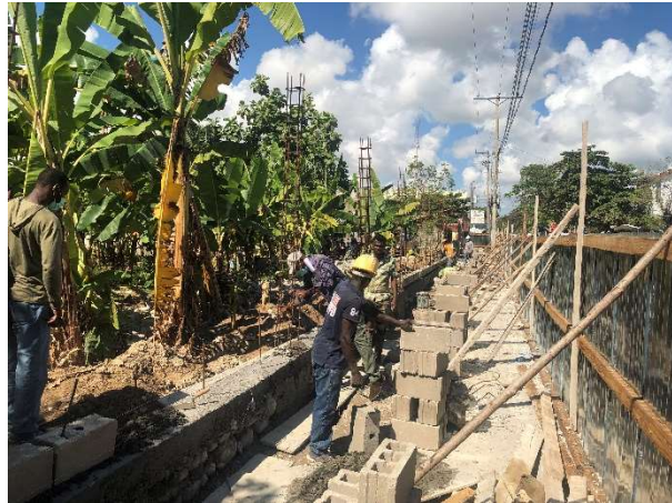
Figure 1. Perimeter wall under reconstruction.
